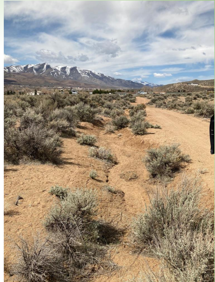
Photo of existing nature create drainage crossing property from NE to SW
